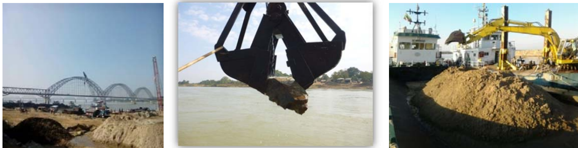
Figure 3. Operations of dredging work and removing snag rock [1]
